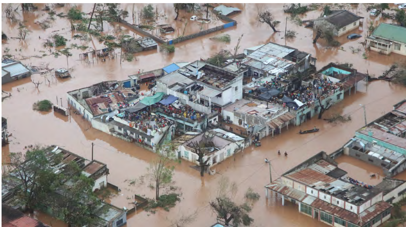
People take refuge on roofs following flooding caused by Cyclone Idai in Mozambique. Credit: World Vision
