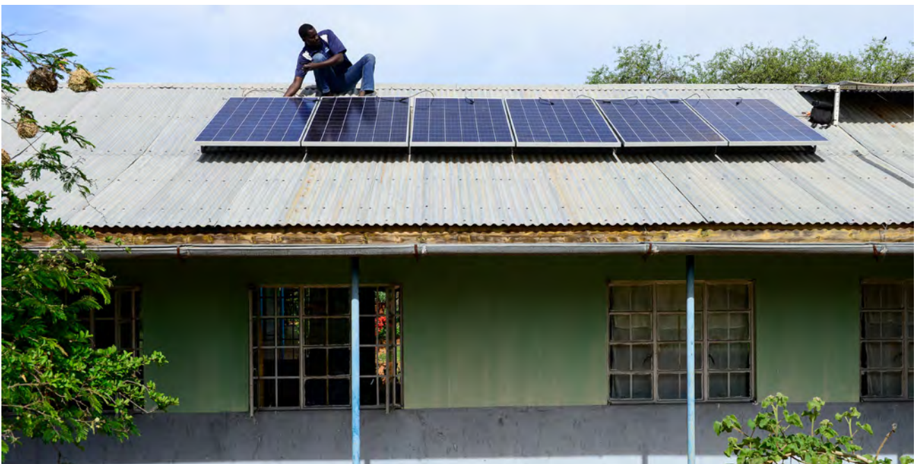
Installing solar panels on a Karamoja house, Uganda. © Joerg Boethling/Alamy
