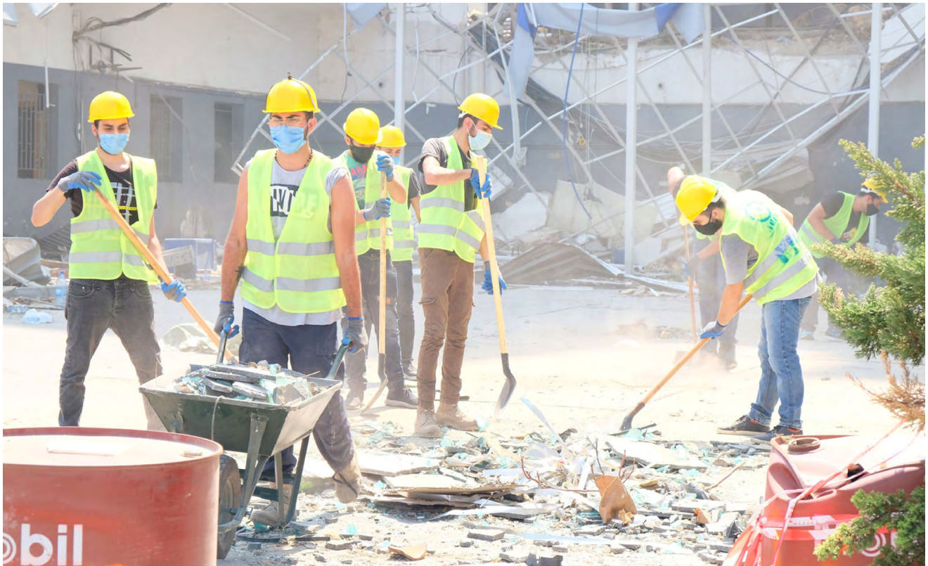
ILO's Employment Intensive Infrastructure Programme (EIIP) creates 200 decent jobs for Lebanese nationals and Syrian refugees to help restore livelihoods and support the clear-up operation in Beirut. Credit: ILO
