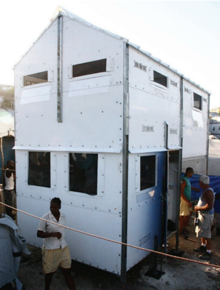
Figure 2 Two-storey shelter in Haiti
