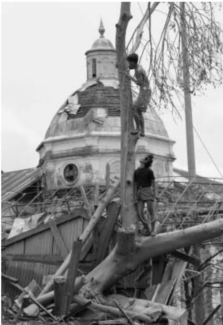
Cyclone damage in Yangon
