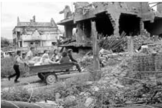
Widespread destruction prompted a massive international response
