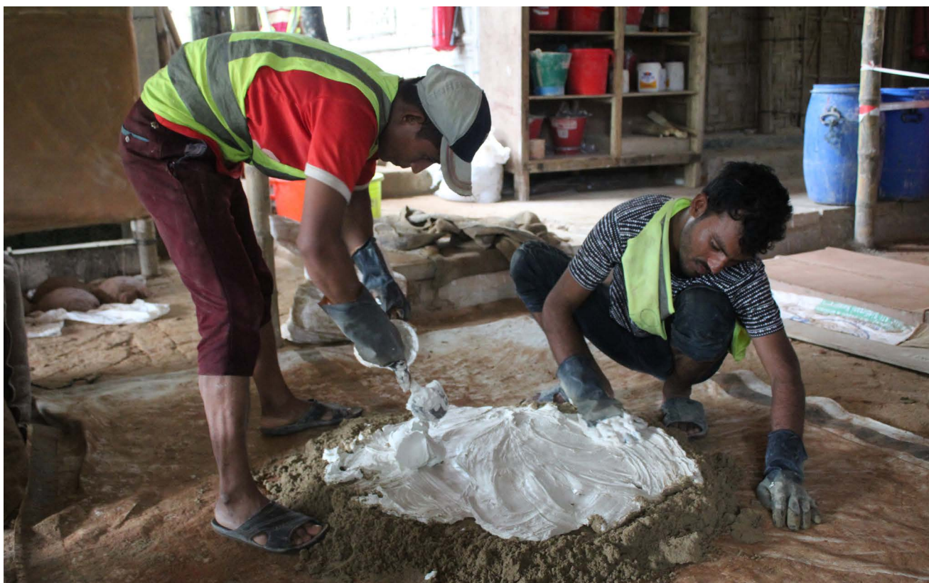
Mixing lime, soil, and other natural materials to create a fire-resistant and durable plaster for shelter construction in refugee camps. Credit: Abdu Sukkur Bappy
