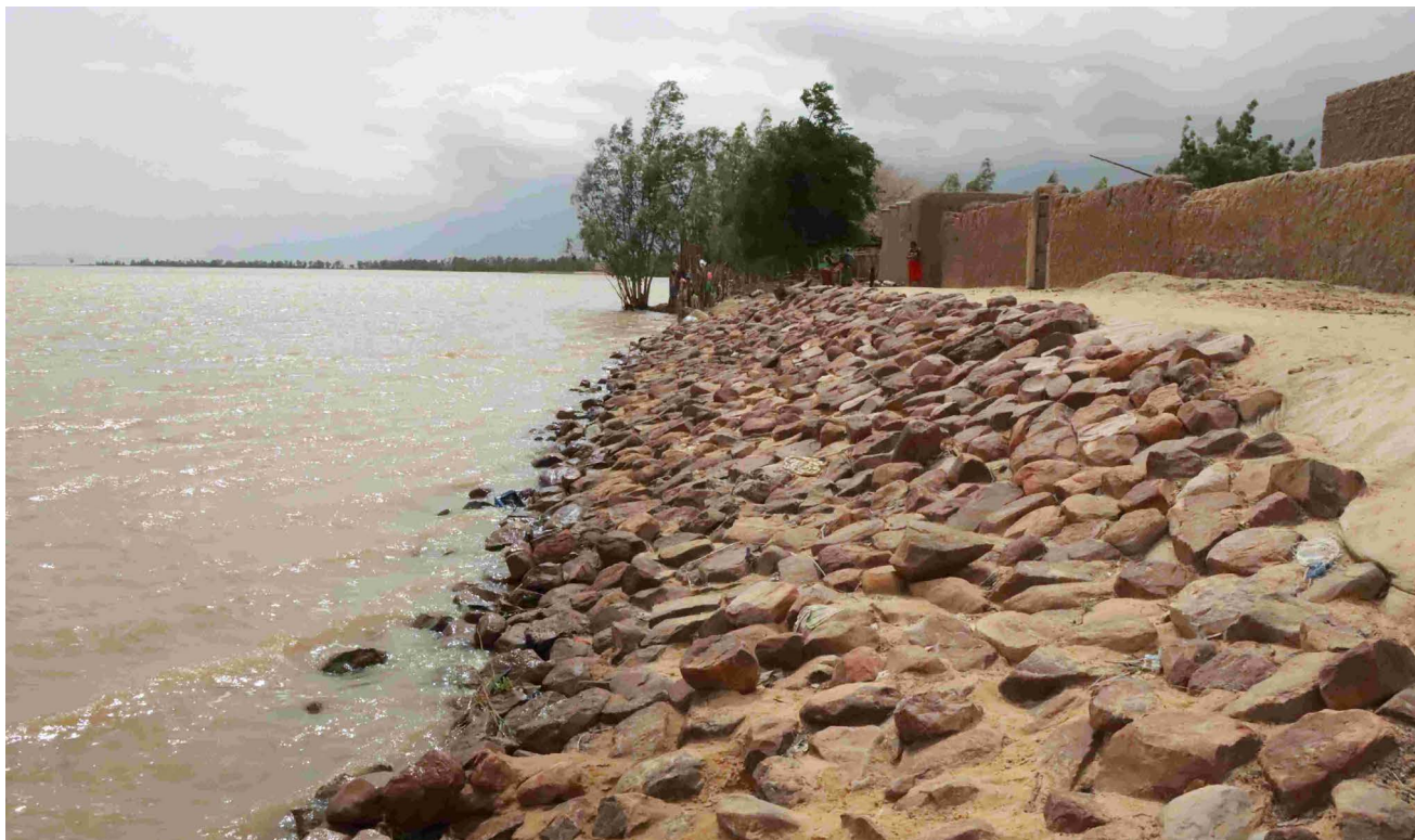
Local populations are raising awareness of the effectiveness of building dikes, using a mixture of banco earth and stone, to protect their villages from floodwaters. Credit: International Medical Corps Mali
