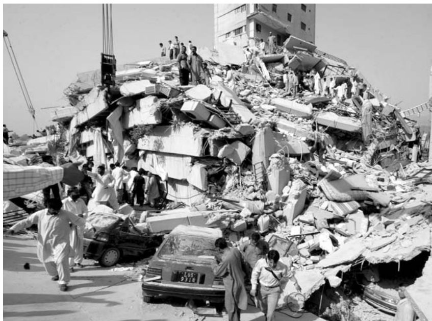
A damaged building in Islamabad, 8 October 2005
