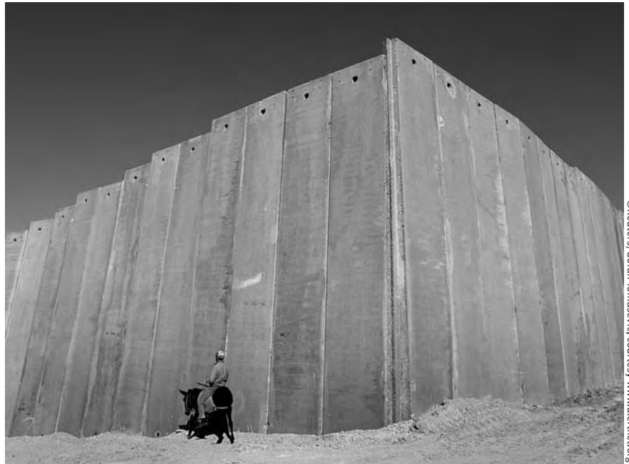
Part of the Israeli separation barrier on the outskirts of Jerusalem
